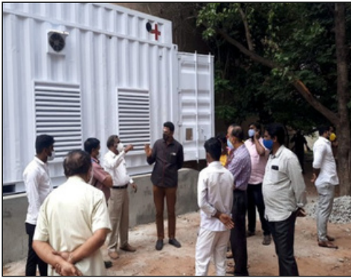
Government Hospital, Chinthamani
